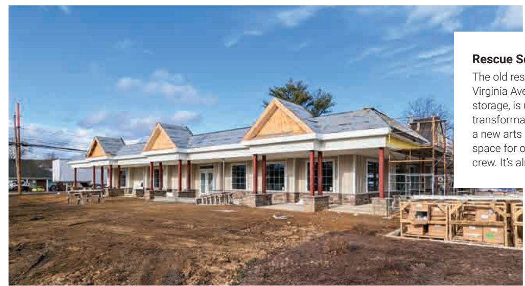
Hearthstone Manor Work began in 2022 to update Hearthstone Manor's curb appeal with all-new siding, a redesigned portico, and new windows and roofing.
